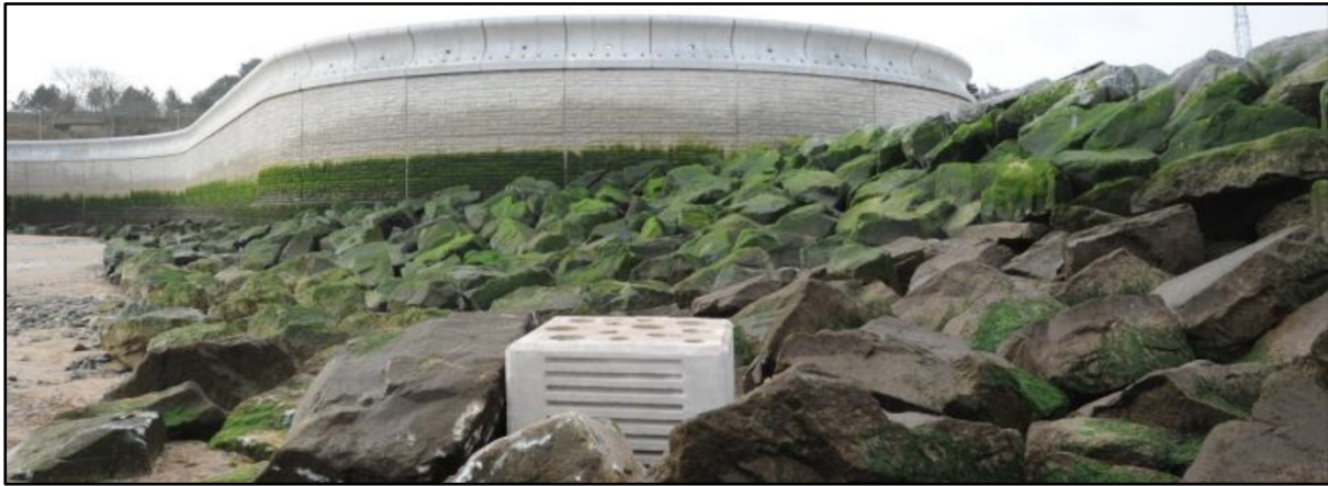
Figure 7. Bioblock positioned within rock armouring at Colwyn Bay (Conwy)
