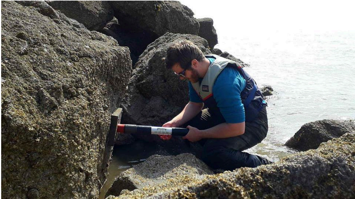
Figure 5. Alternative concrete tile being fitted at Mornington, Meath (Ireland) as part of the Ecostructures project
