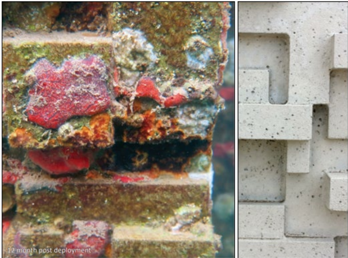
Figure 4. ECOConcrete® sea wall tile deployed at Herzliya Marina, Mediterranean Sea (Israel)
