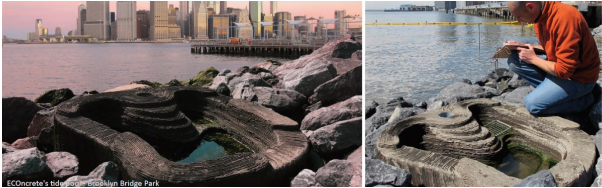
Figure 23. Tide pools installed amongst rock armouring/rip rap in New York (US)
