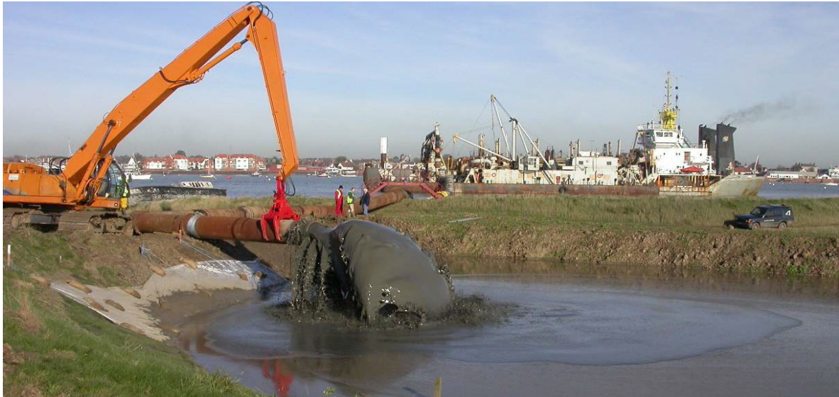
Figure 11. Large-scale (550,000m 3 ) beneficial use of dredged silt for pre-breach land forming at Allfleet's Marsh on Wallasea Island (Essex, England)
