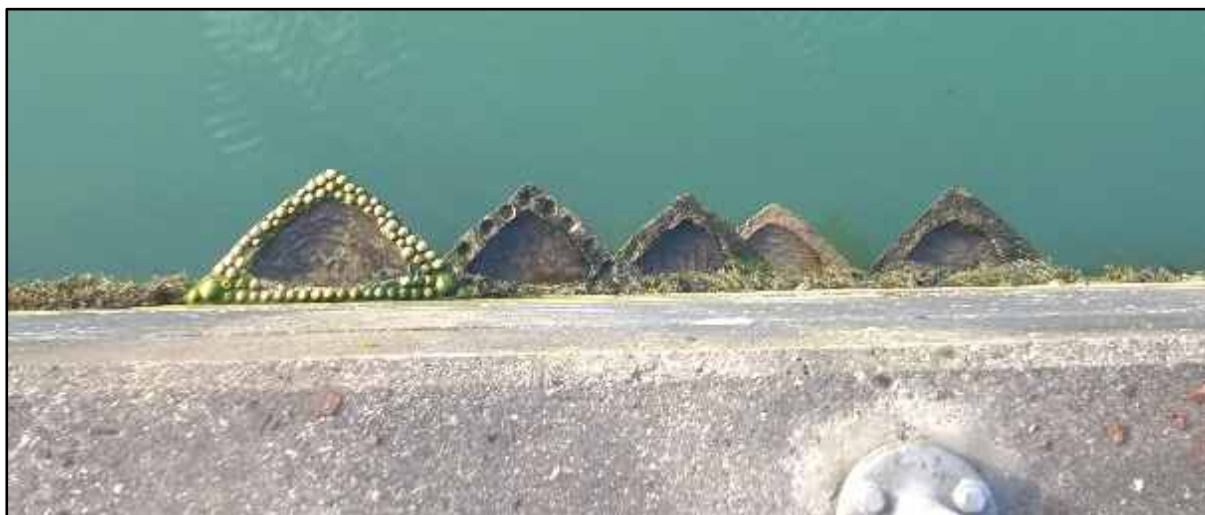
Figure 2. 'Vertipools' at Fishbourne (Isle of Wight, England) (two months after installation)
