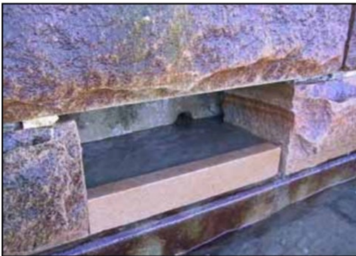
Figure 21. Artificial pools in a vertical sandstone wall, Sydney Harbour (Australia)
