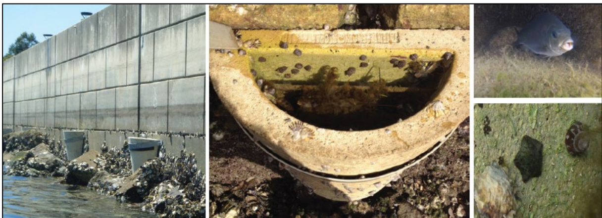
Figure 20. Custom-made ‘flowerpots’ retrofitted to Sydney Harbour (Australia) seawall (close up of cushion star and luderick fish found in some pots on right)
