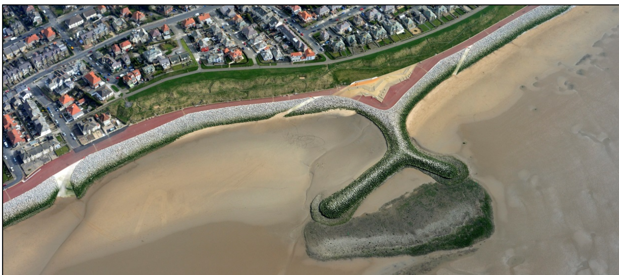
Figure 26. Breakwater at Morecambe (Lancashire, England) with innovative rocky habitat mitigation area in front
