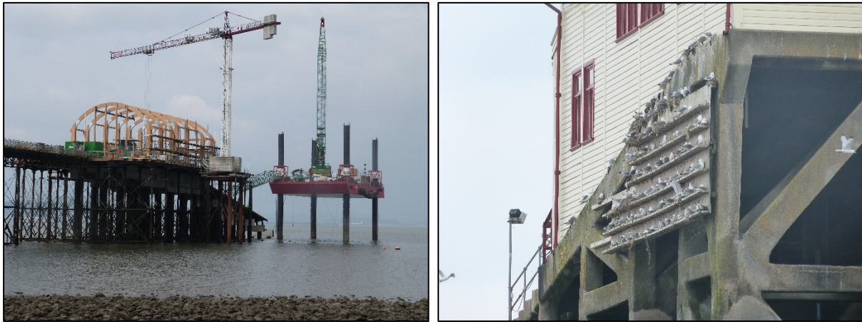
Figure 15. Pier development at Swansea Bay and site enhancement through placement of Kittiwake nesting platforms at Mumbles Pier
