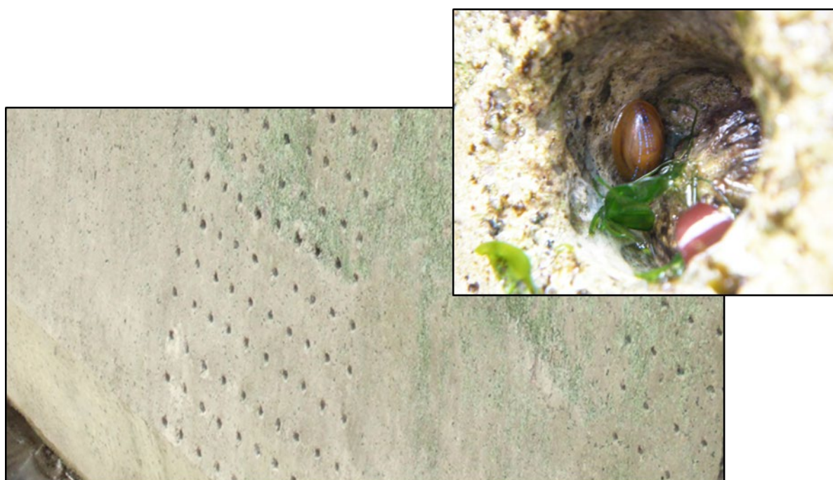
Figure 3. Drilled sea wall at Sheldon (Devon, England) – inset shows limpets and red and green algae occupying one of the drilled pits
