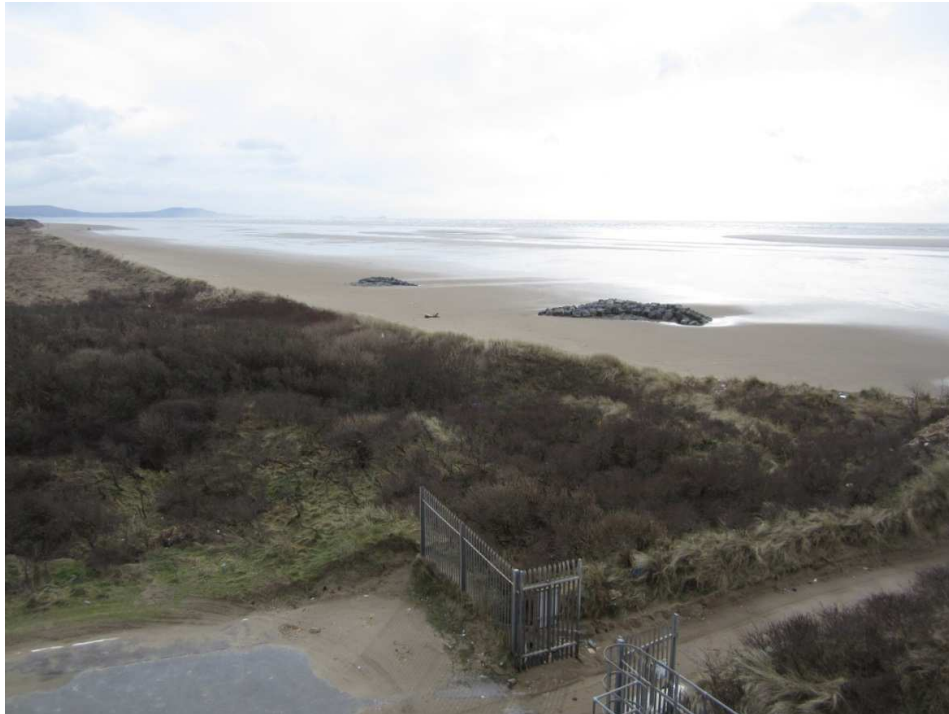
Photograph 9: Rock armour protection near the Pembrey Sands control tower; view looking southwest.
