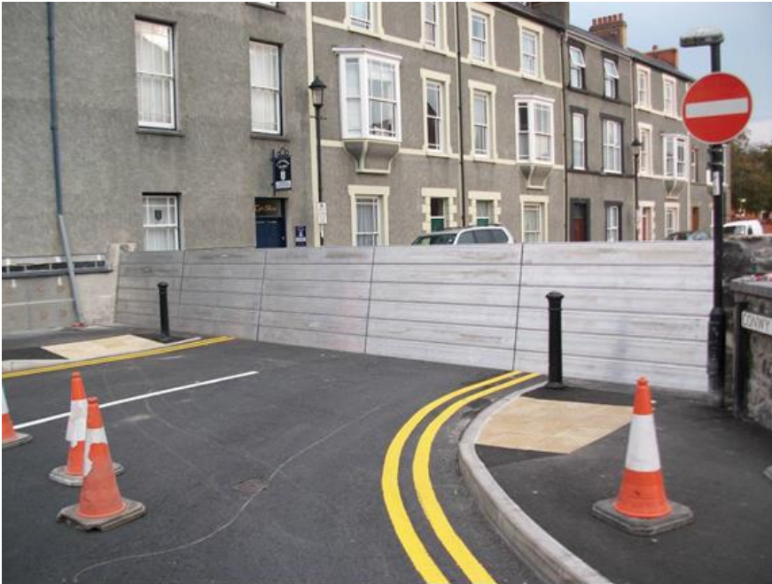
Figure 4 - Conwy Terrace Demountable Defence
