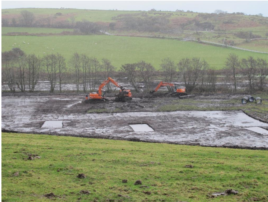
Figure 22. Peat stripping work in progress at Cors Ceidio in February 2014 as seen from the lane at the top of the slope to the NW of the site (see Fig. E for location). The three flooded oblong areas are deeper excavations designed to mimic historic peat cuttings which remain a short distance to the right (SW) of this image. The new access track to the opposite (E) side of the fen is seen to the right in the distance.
