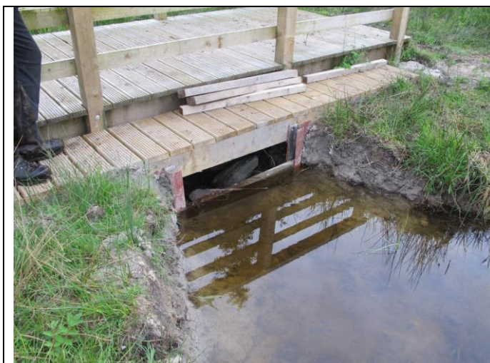
Figure 5. The main drain sluice at Cors y Farl installed by LIFE contractors A.J. Butler and Matt Sutton in spring 2013. Alder weir boards are visible stacked on the boardwalk ditch crossing beside the stock-bridge.
