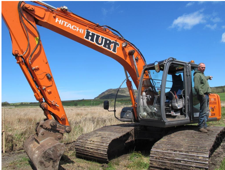
Figure 11. 360 degree Hitachi excavator fitted with 1.2 m wide tracks. This or similar machines were used at Cors Cefn Uwrch, Mathan Uchaf, Cors Bodeilio and Cae Gwyn for peat stripping and hydrological restoration projects.
