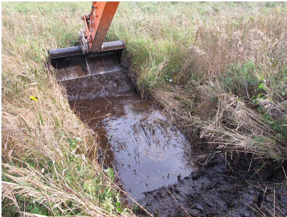
Figure 7. Excavation of a notch in a ditch line running left to right. The notch is recessed into solid peat either side of the drain to act as a 'key' for the peat dam.
