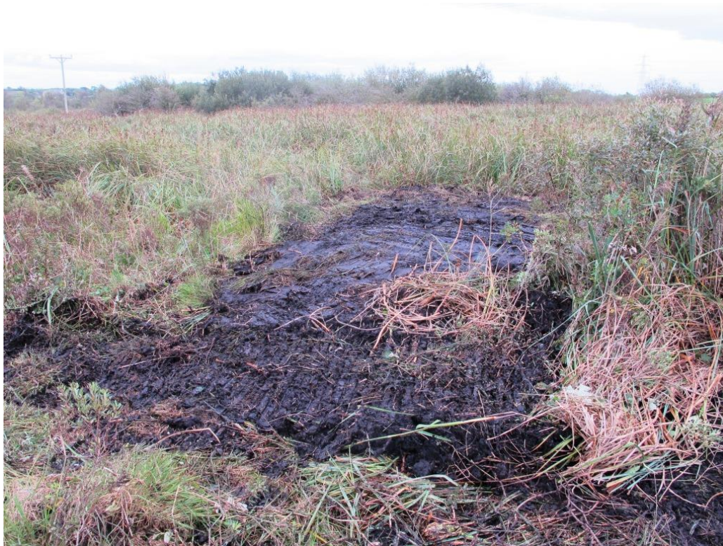
Figure 8. Completed peat dam perpendicular to the left to right axis of the drain. Note the thickness (left to right in this image) of the dam.
