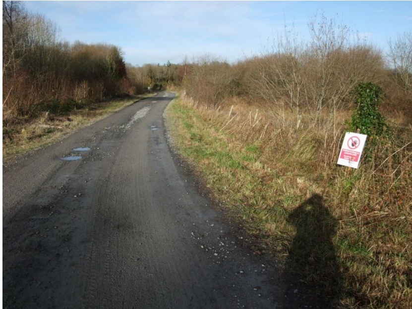
Fig. 1: Site 1J, 17.12.2013 - Trackside (looking NNW)
