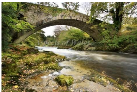
Pont Dolauhirion, Afon Tywi
