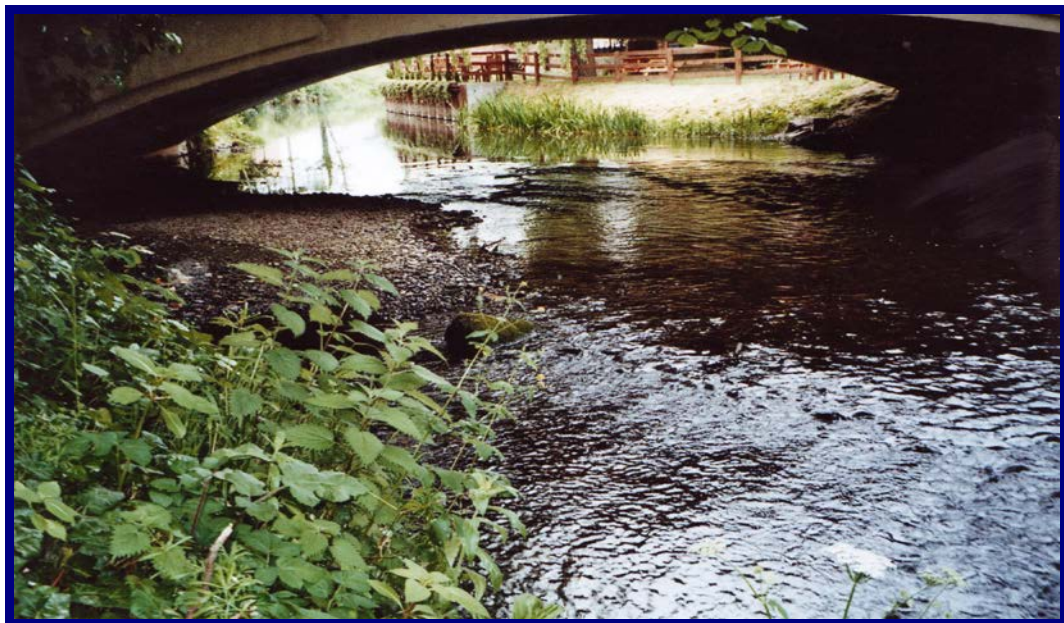
Picture No. 9 – The same River Alyn bridge at Rossett looking upstream showing the 42” of silt which has not been removed.
