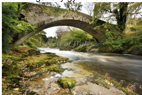
Pont Dolauhirion, Afon Tywi
