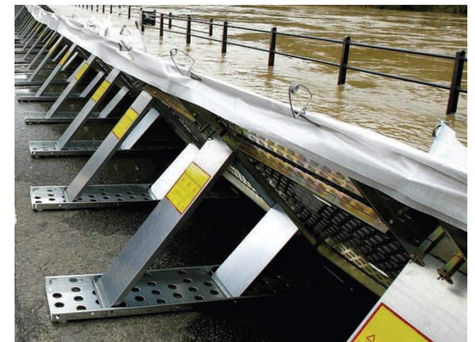
Temporary defences in operation . (Environment Agency)
