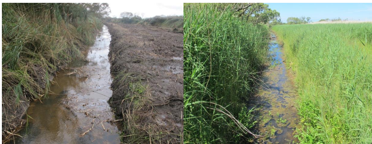
Figure 3. The main ditch at Cors Hirdre upstream (W) of the plank bridge close to dipwell DWM9. The L image (30/8/13) shows the ditch immediately after being cleaned, the R image shows the same location on 16/6/14: note the significant reed growth through the spoil (all of which was deposited on the N bank at this location) and also dam D3 in the distance of the RH image.
