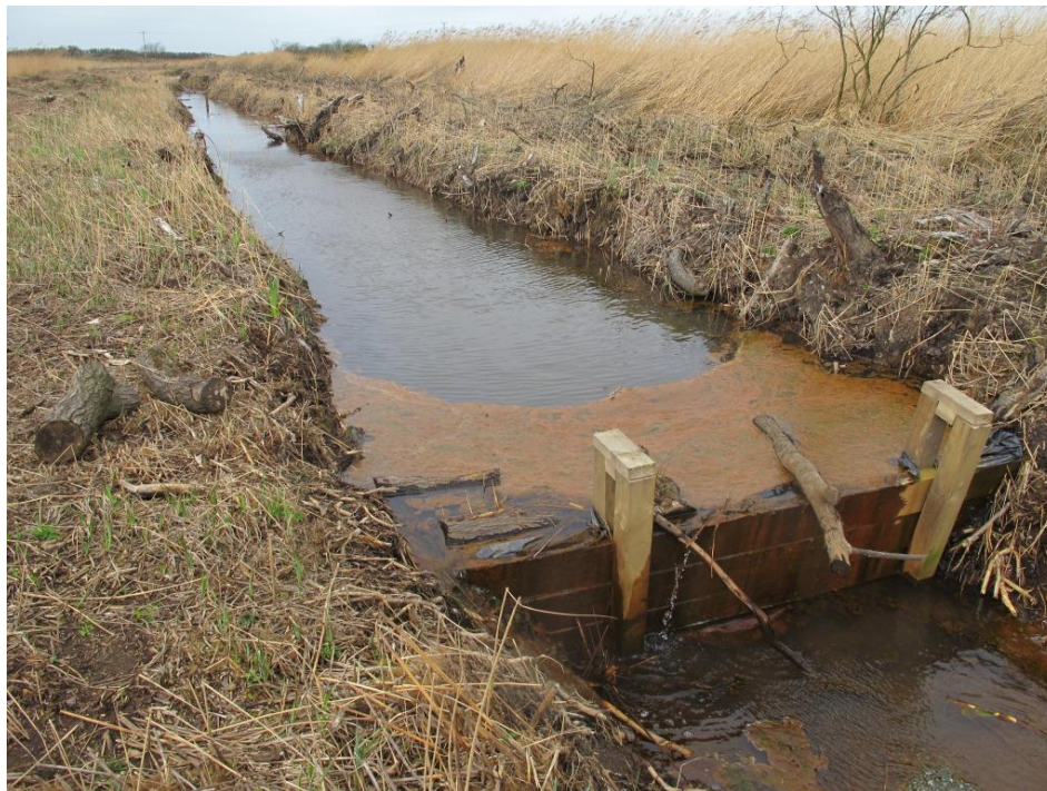
Figure 18. Water levels in the recently cleaned main drain upstream of Dam D2, 19 March 2014. The water level upstream of the dam is probably slightly above the base of the peat in this image, this is the recommended level.
