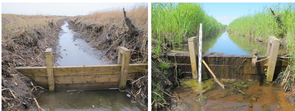
Figure 4. View of dam D2 looking upstream on 6 February 2014 (L) when dam leakage was resulting in similar water levels both up and down-stream, and 13 June 2014 (R ) following measures to line the dam. The dam is sustaining a water level difference of 48.2 cm upstream (water level at dam crest) and downstream of the dam in the R hand image.
