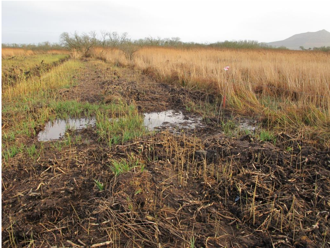
Figure A.3.5. Looking east along S side of recently cleaned ditch with dipwell DW5 flagged to right. A channel (flooded) has been left in the spoil bank by the digger operator.
