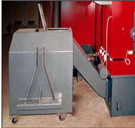
Automatic ash removal from the boiler
