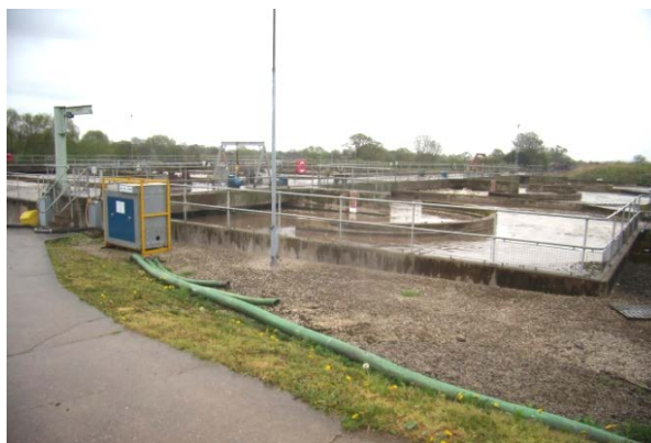
Five Fords waste water treatment plant
